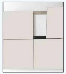
**Step-3**:- First Merino HPL compact panel is completely mounted, second Merino HPL compact panel is getting mounted on the profile.
